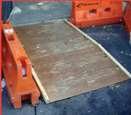
Figure 21: This temporary curb ramp is at a low grade, utilizes non-slip materials (e.g., non-slip coated wood), and is wide enough for ADA-compliant access. Temporary curb ramp solutions are still an area in need of further innovation.
