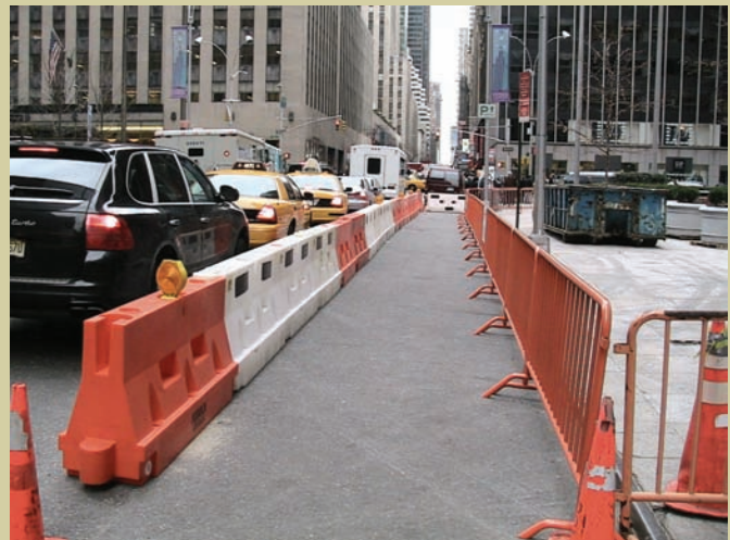
Figure 11: Physical separations must shield pedestrians from construction and traffic. This walkway setup includes brightly-colored barricades with reflectors and brightly-colored metal fencing, providing a wide, set back walkway that is adequately guarded from both street traffic and construction activity. However, the fencing is not ADA-compliant due to a lack of a lower rail for walking canes and the tripping hazard caused by the supports protruding into the walking way.
