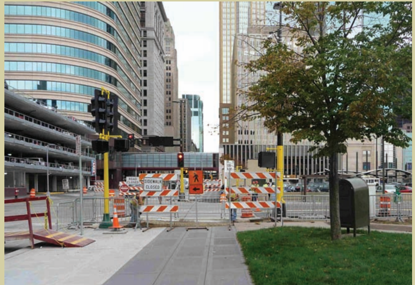
Figure 16: These signs provide adequate information to alert pedestrians that the sidewalk is closed and to use the alternative path defined by barricades and channelizers, and includes an ADA accessible ramp due to the steep grade change from sidewalk to street.
