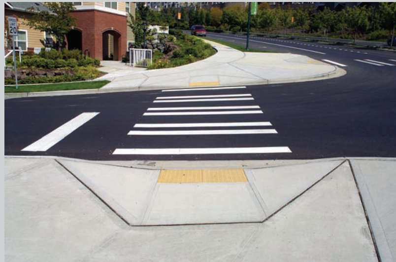
Figure 46: This Bar Pairs Crosswalk is highly visible due to the breaks between striping, alerting drivers that they are approaching a crosswalk.
