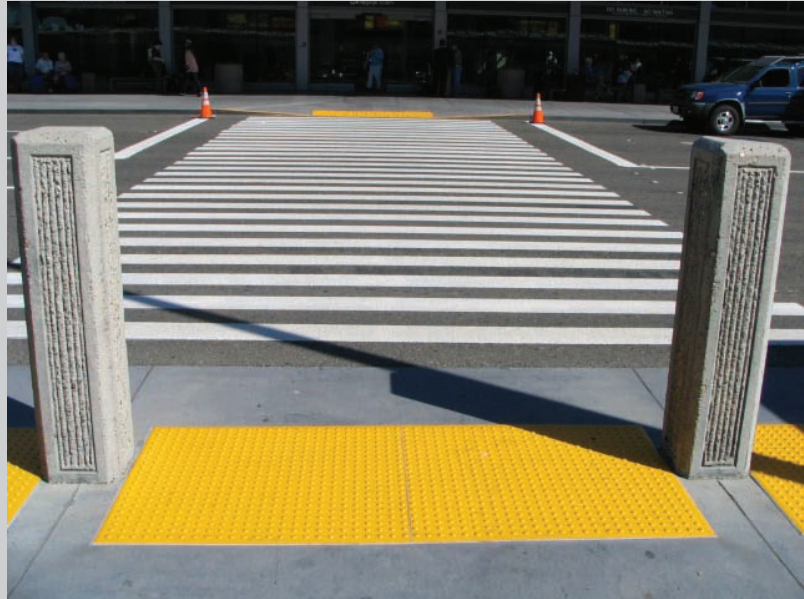
Figure 45: This Continental Crosswalk includes brightly painted striping and is also accompanied by ADA compliant curbs and concrete barriers to warn pedestrians to cross within the crosswalk.
