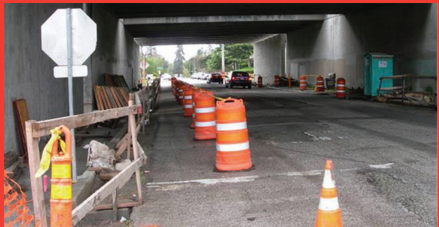
Figure 23: This detour is a common example of an ADA non-compliant work zone pathway. The drums do not provide sufficient protection from traffic, are not continuous, and the pathway is not wide enough to accommodate wheelchairs or carts, and the pathway is dark and unlit.
