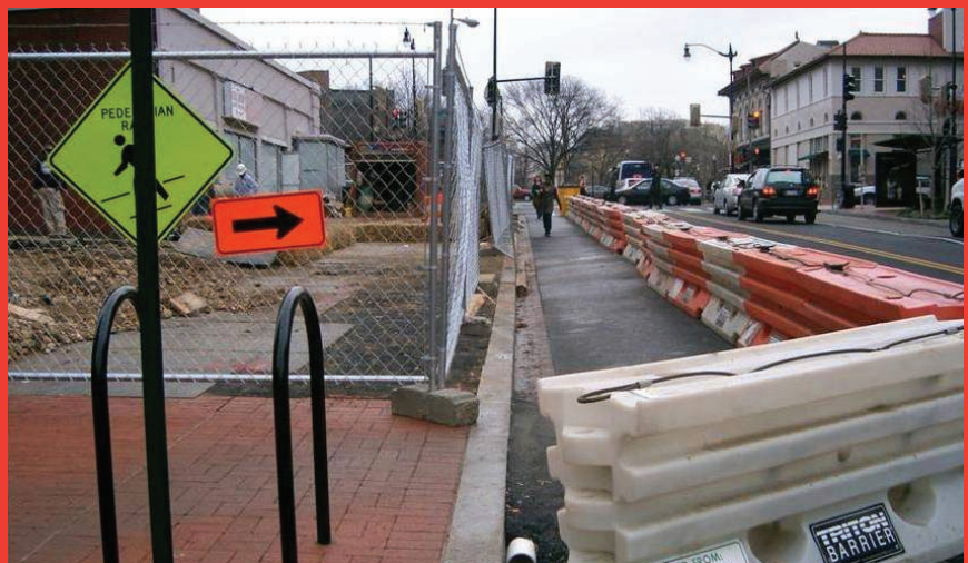
Figure 22: This work zone detour provides a solid barrier to traffic through the use of longitudinal channelizers, is an ADA accessible width, and incorporates a low-grade curb ramp.
