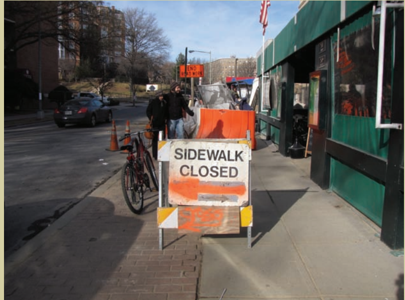
Figure 15: This vertical construction zone is missing proper signs to guide pedestrians to a safe crossing or diverted pathway. This sign is defaced and altered to be non-MUTCD-compliant. Additionally, it improperly directs the pedestrian to cross at an unsafe crossing area devoid of a crosswalk.
